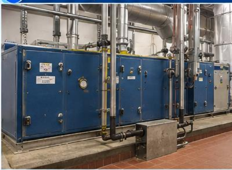
7 Air Handling Unit (Actual Unit)
